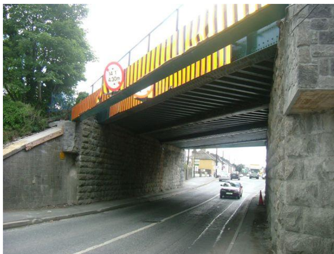
Plate 25: Advance structure – collision protection beam
