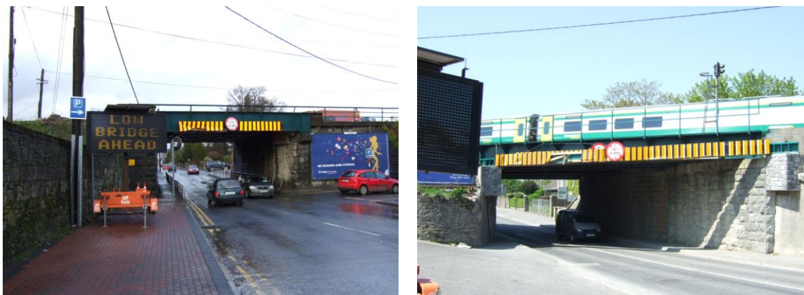
Plate 7: Portlaoise Under-bridges, UBC145 (left) and UBC146 (right)
