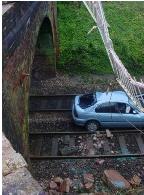
Plate 32: Over-bridge strike and debris on the line
