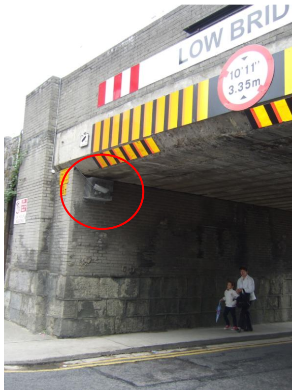
Plate 31: CCTV Surveillance at Restricted Bridge No. 107, South Lotts Road
