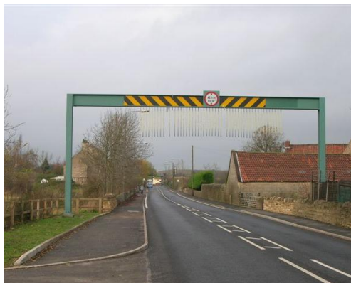
Plate 24: Hanging chain (GB) and bell (Korea) arrangements
