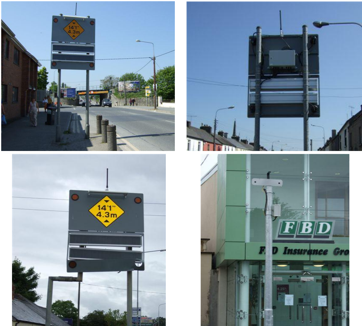
Plate 29: Infra red detection equipment installed in Portlaoise
