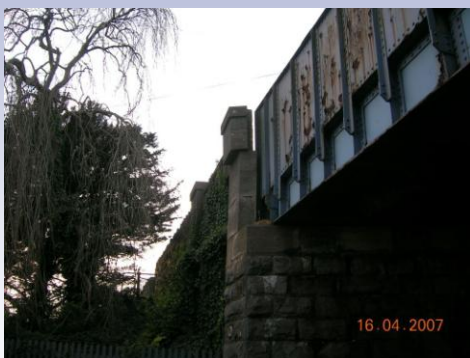
Wrought Iron Parapet
