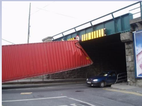
Steel beam bridge
