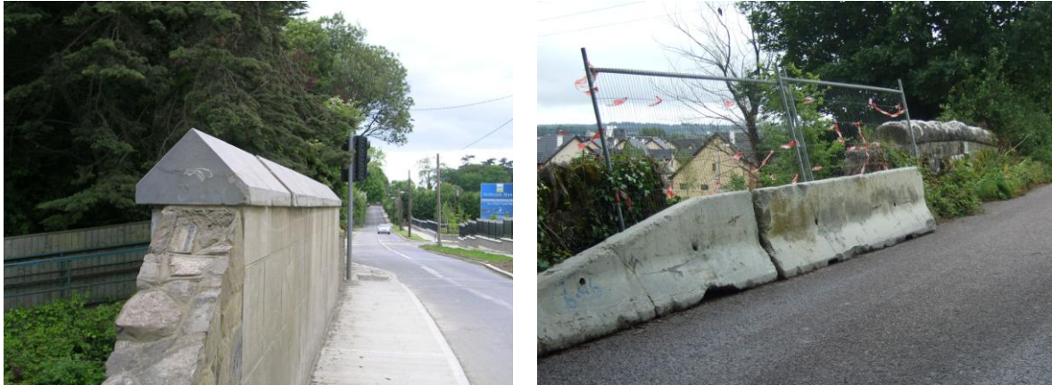
Plate 6: Examples of Masonry over-bridge damage
