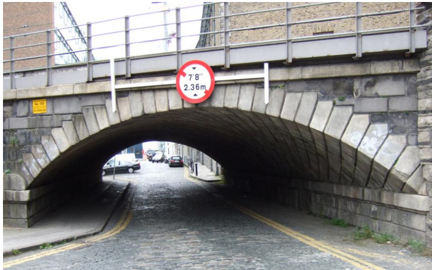
Plate 21: Masonry arch under-bridge with goal-posts.
