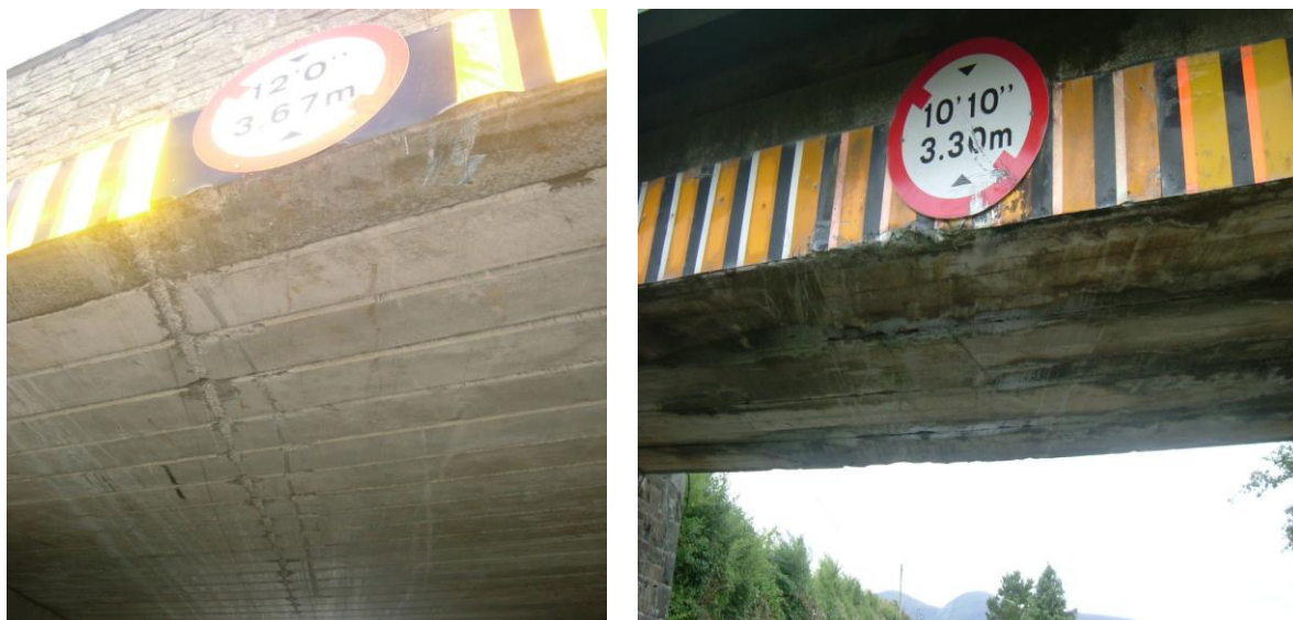
Plate 5: Superficial damage to concrete under-bridges
