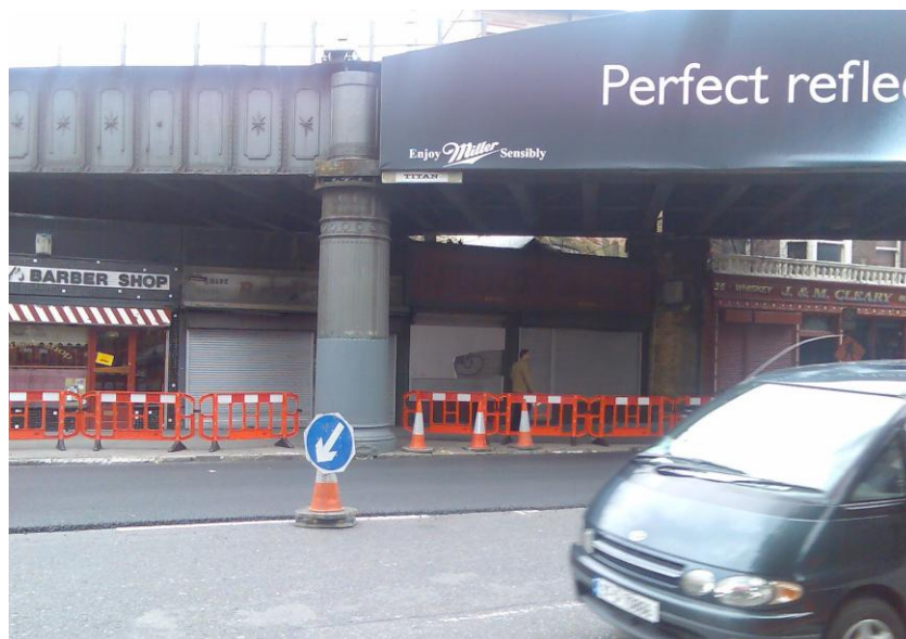
Plate 22: Road Surfacing under a height restricted bridge
