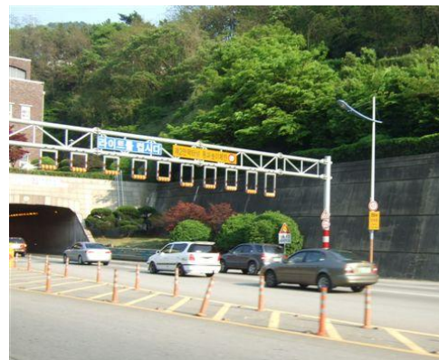
Plate 24: Hanging chain (GB) and bell (Korea) arrangements
