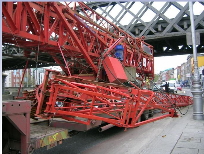
Wrought Iron Lattice/Truss
