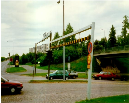
Plate 23: Portal frame on the approach to a headroom restricted bridge
