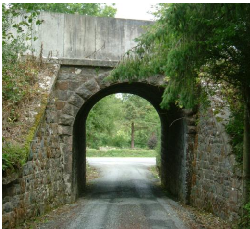
Masonry Arch
