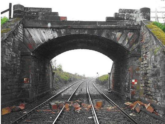
Plate 2: Examples of an over-bridge strike
