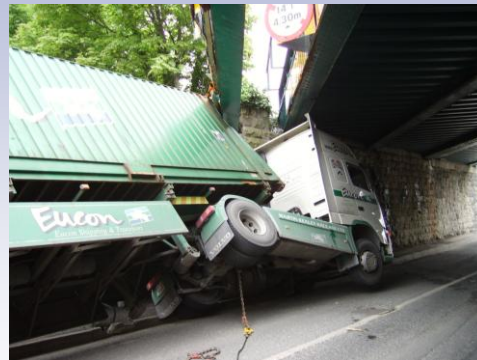
Steel beam bridge with bash beam
