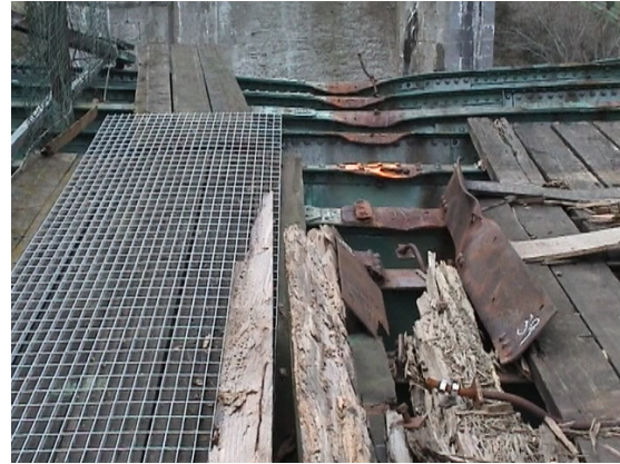
Figure 13 Detail of Down side after debris was removed
