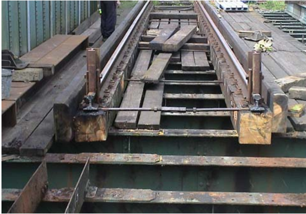
Figure 9 Way-beams over transverse girder 18
