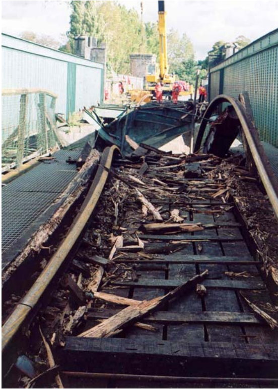
Figure 12 View of collapsed deck from Limerick side of Viaduct
