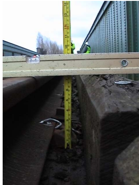
Figure 24 Height of rail above guard-beam at Way-beam 6
