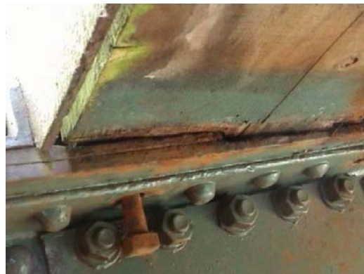
Figure 26 End of Way-beam 6 at transverse girder 21
