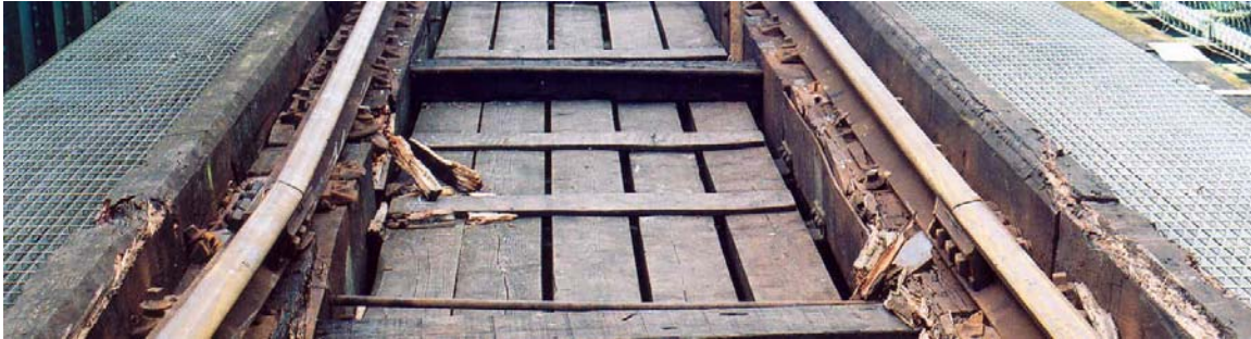
Figure 14 View of secondary deck, looking back toward point of original derailment
