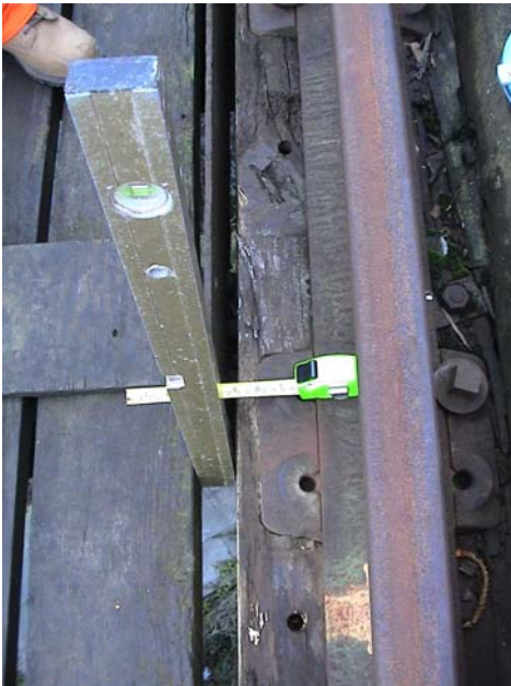
Figure 23 Outward tilt of way-beam 6
