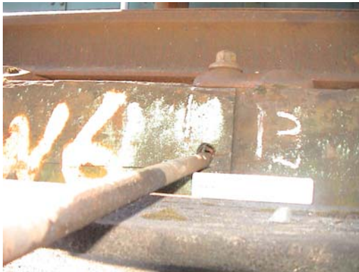
Figure 25 Tie-rod hole elongation on way-beam 6, between transverse girder 15 & 16
