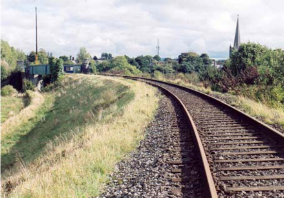
Figure 6 Viaduct from Limerick side
