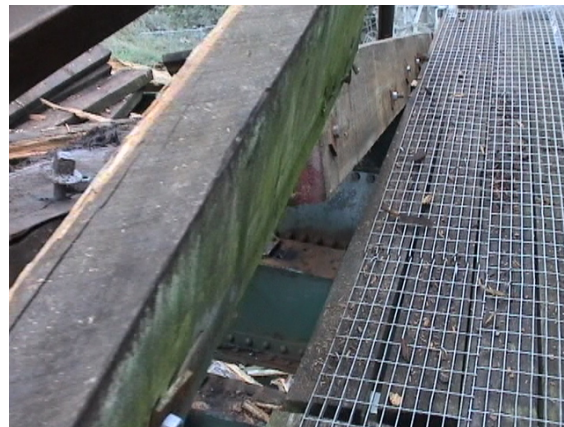
Figure 20 Up guard-beam and decking arrangement
