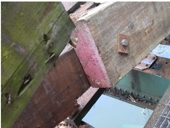
Figure 18 Old guard-beam abutting new guard-beam on Up side: way-beam behind has deep notching at its base
