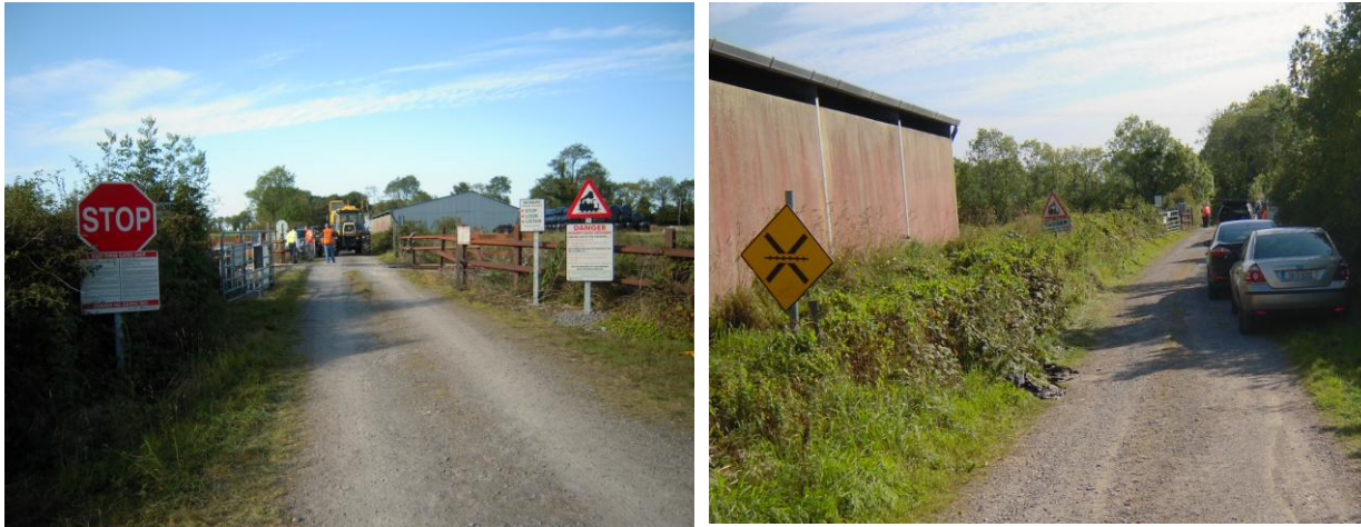
Figure 1: Signage at XM096 – South of railway line (left) and north (right) Photos taken -2 nd September 2010)
