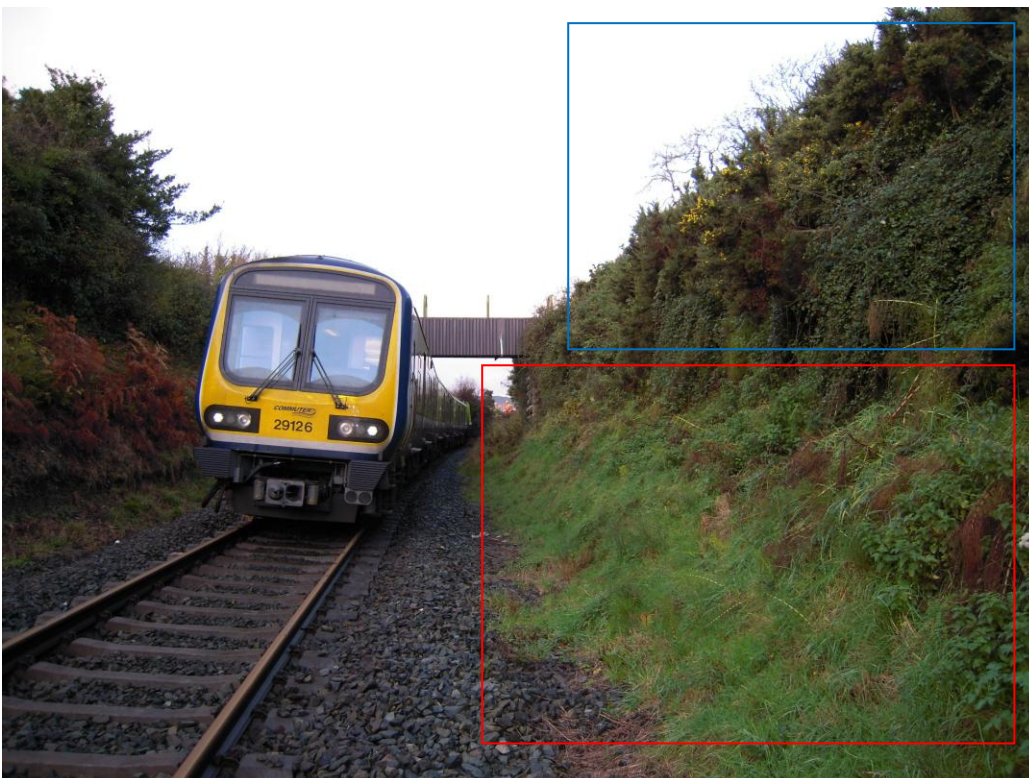
Image illustrating the vegetation above the reach of the flail (blue) and in the reach of the flail (red).
