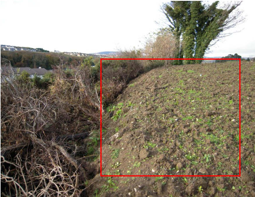
Photograph of field showing 'surcharging' or deposited soil at cutting top.
