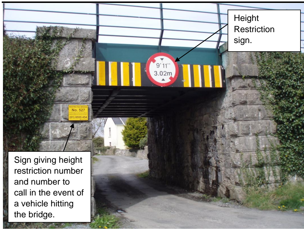
Figure 11 Height Restriction Signage on Bridge under Railway
