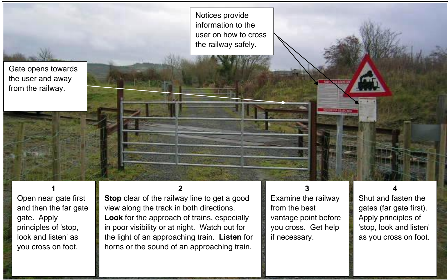
Figure 6 Iron Gated Crossing on Road (unattended)
