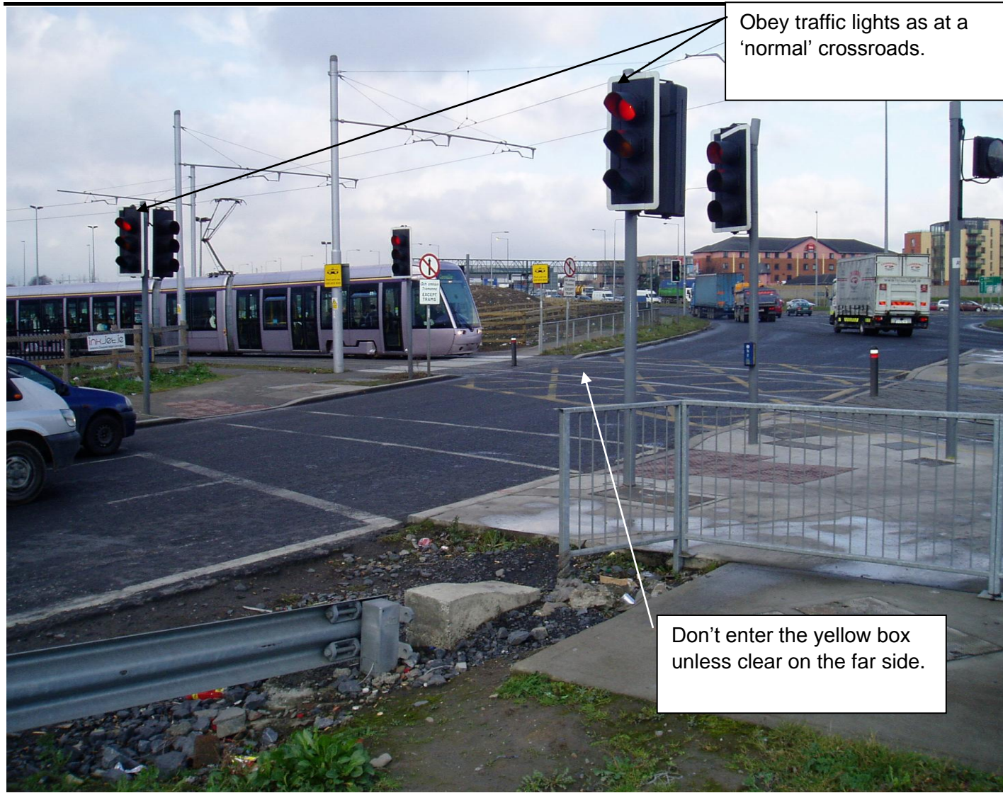
Figure 10 Road Intersection with Tramway Crossing
