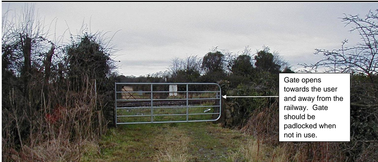
Figure 7 Iron Gated Crossing (Field)
